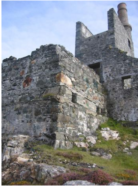
Nineteenth Century Mine pumping engine in Cornish style (Allihies).
